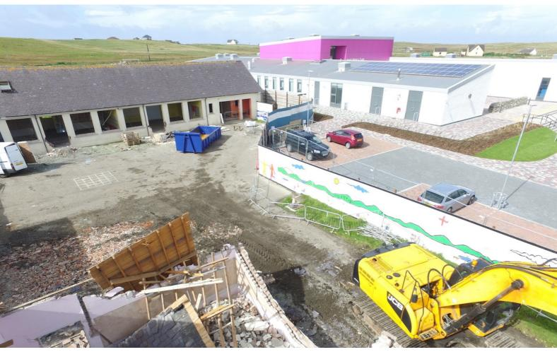
MAL carried out on-site crushing of all masonry material recovered from the demolition works. The recycled masonry was reused in the reinstatement of site.
