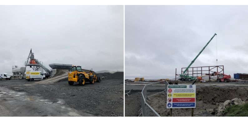
MacAulay Askernish Ltd (MAL) provided in-house resources to carry out all Civil works, utilising local labour and material. MAL carried out the on-site wet concrete batching of 4000m3 used in the construction of hardstanding's, Blast Wall, Concrete Roof and Floor Slab. Also supplied was over 15,000 tonnes of infill material for the project. All raw materials with the exception of the cement were sourced on Island.
